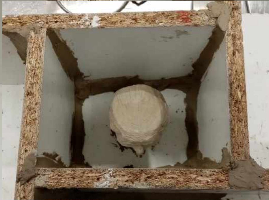
STEP 1 - BUILD A WALL USING WOODEN BOARDS AND THEN USE CLAY TO CLOSE THE GAPS.
