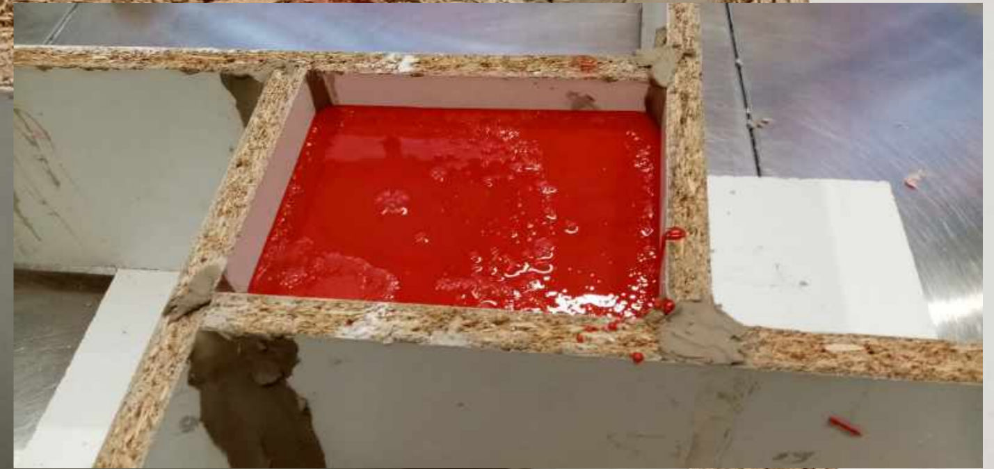
STEP 2 - POUR MELTED VINYL INSIDE THE WALL AND LEAVE TO SET.
